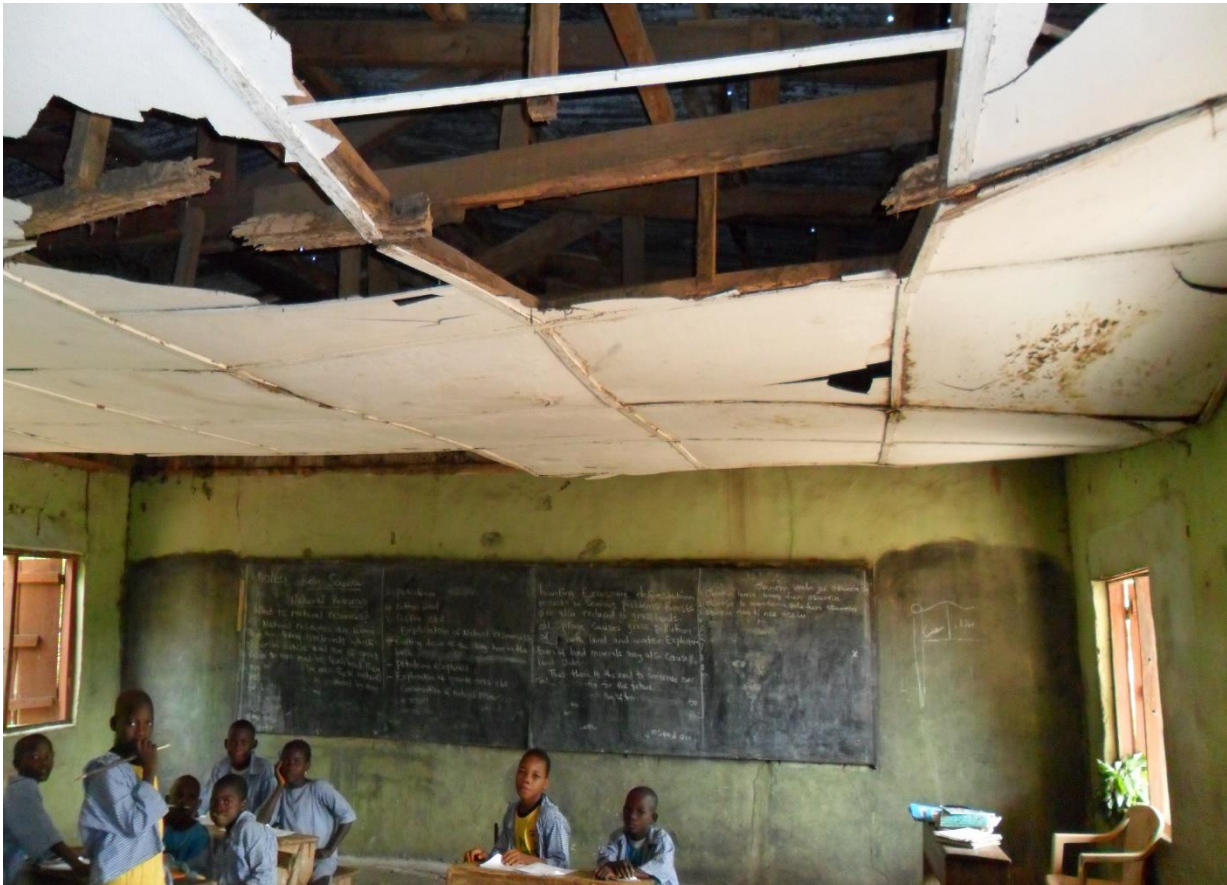
Figure 9: Collapsing roof of a classroom.
